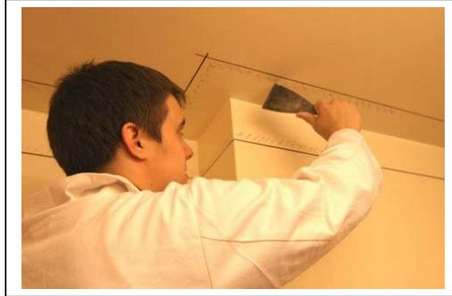
Start to fix at the most visible point in the room. Typically the external mitres on a chimney-breast are a central feature and should be used as the starting point. Work away from the most visible point in both directions left and right towards a corner of the room that is less obvious, for example above the entrance door. This mitre will be less noticeable if there is a difficulty with pattern match towards the end of the fixing procedure.
