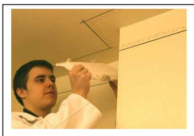
*For extra security the cornice should then be mechanically fixed with zinc plated screws at 900mm centres through every other dab of adhesive and into ceiling joists were possible*
