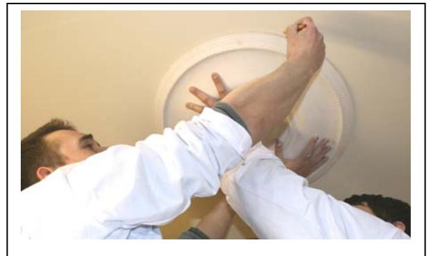
3. Using a bradawl, probe within the marked area and locate the ceiling joists.
