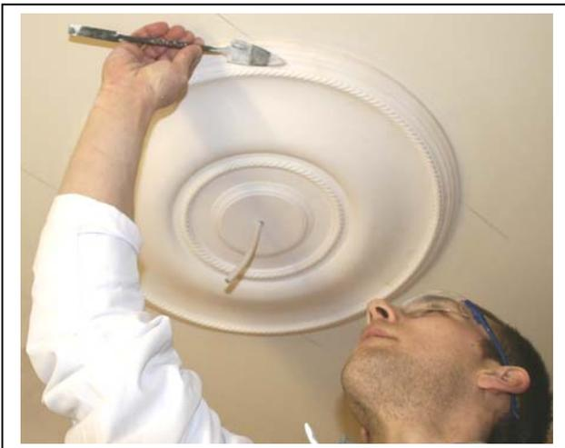
*When pointing and filling, it is recommended that the area be lightly dusted with a damp brush to control suction and setting time of the filling/pointing material.*
