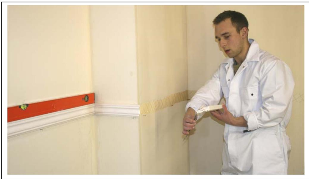
If the dado rail is to go up a stairway, measure the required height for the rail at right angles to the stairs from the front of the treads at the top and bottom of the stairs, then use a chalked line between these marks to set the line for the rail up the stairway - extend the line to intersect the marks for the horizontal rails at the upper and lower floors.
