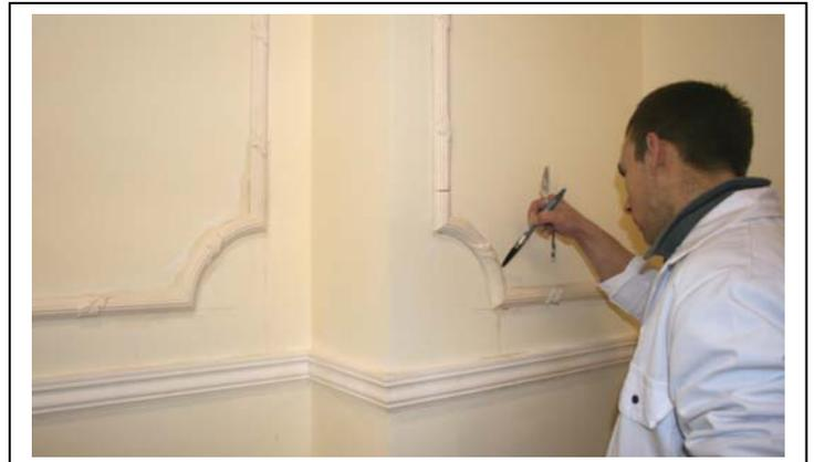
4. When pointing and filling, it is recommended that the area be lightly dusted with a damp brush to control suction and setting time of the filling/pointing material.
